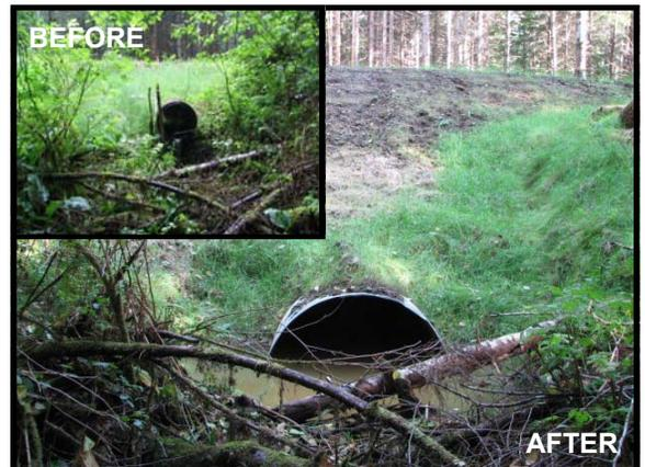
BEFORE and AFTER shots on Smith Creek: One of four culvert replacements in fish bearing streams draining into Smith Creek conducted by Weyerhaeuser Company in Twin Harbors this year. This project replaced an undersized 30" round pipe with a 6' culvert. Both photos were taken in the summer. As you can see, the replacement has repaired the large outfall drop, allowing for adequate passage of salmonids during periods of high flows.
