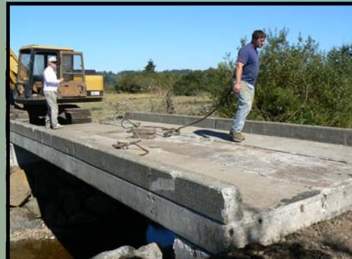
The Vance Creek Bridge Project nearing end of construction. This photo illustrates the bridge slabs that were donated by Grays Harbor County.
